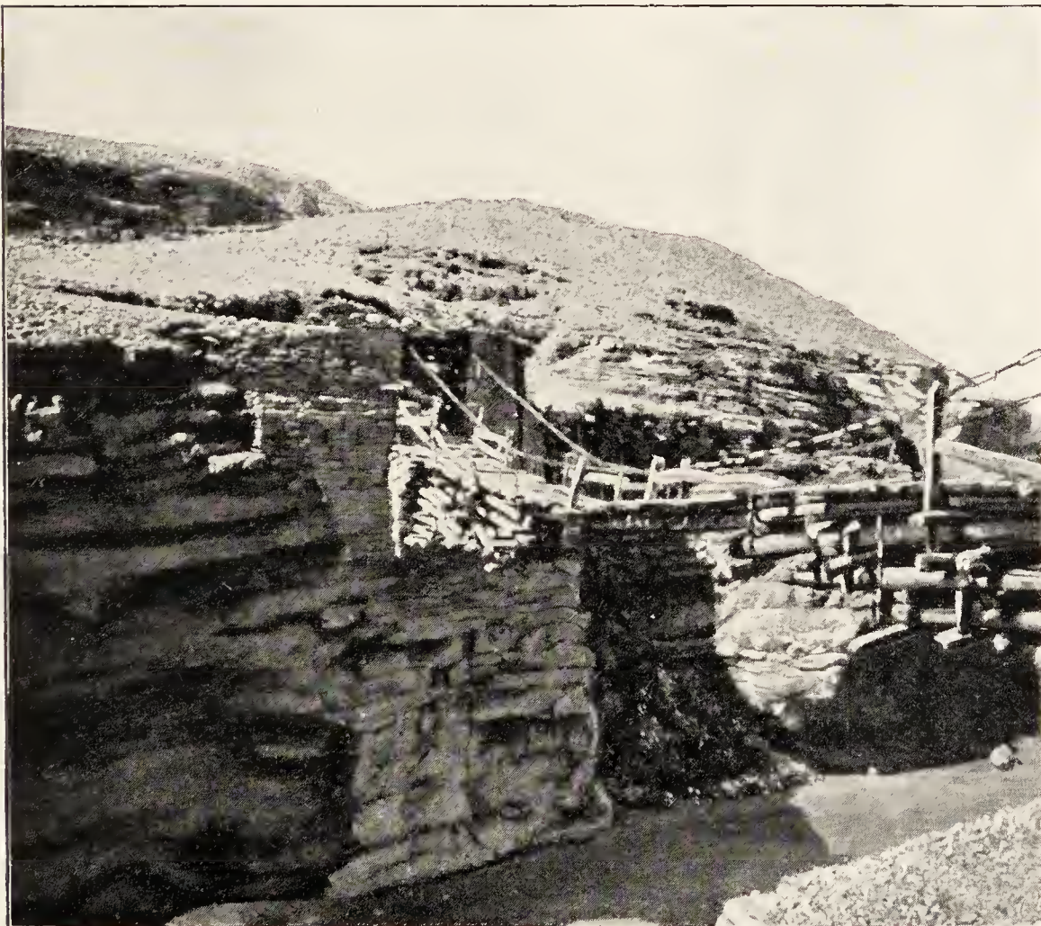
117 AND 118. THE BRIDGE OF TOTLING.
